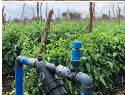
Figures (top to bottom), 3: Layflat; 4: PVC pipe; 5: Blind pipe, connectors, and lateral line; 6: Air valve and filter.
