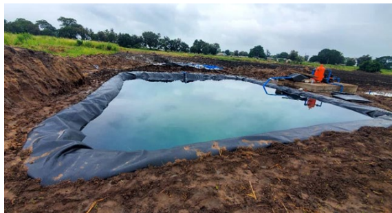
Figure 3: A dam liner retains the water supply for a drip irrigation system.
